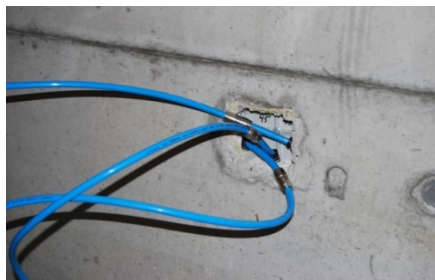
Figure 10: a) Vacuum test/injection hoses,
